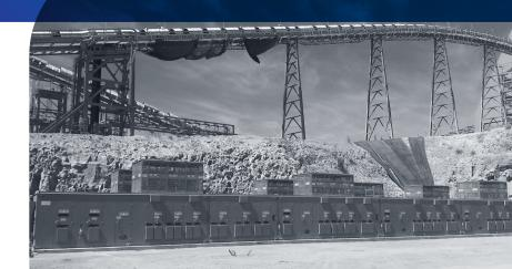
When calculating BIE for electrical components used in mining operations, allowances need to be made for the "derating" effects caused by air conditions at higher altitudes.
